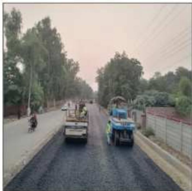
Picture 63: Asphalt base course at Iqbal Road Sahiwal
