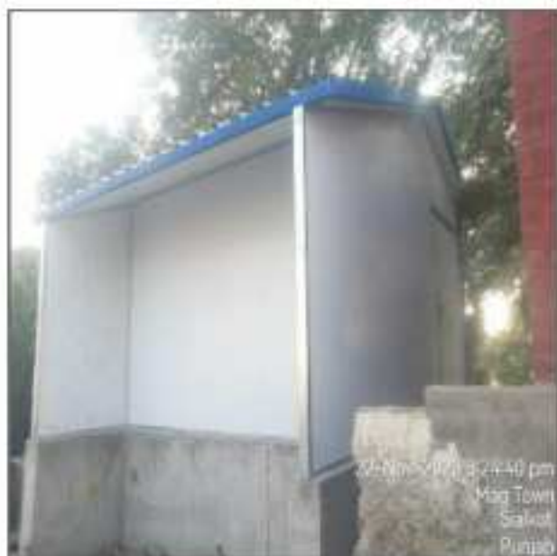
Picture 50: Installation of prefabrication in progress at filtration plant LOT-4 Sialkot.
