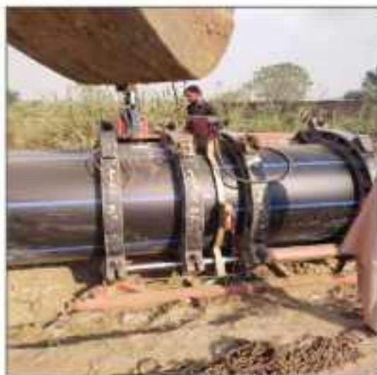
Picture 46: Joining is in progress at Airport Road LOT- 3 Sialkot
