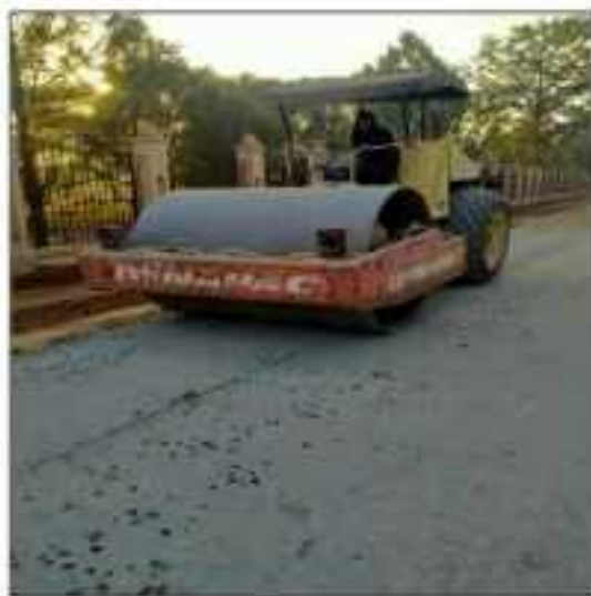
Picture 38: Compaction of WBM is in progress at KSR LOT-1 Sialkot.
