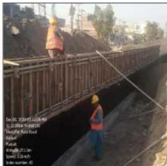
Picture 82: Retaining wall is in progress at flyover site Sialkot.
