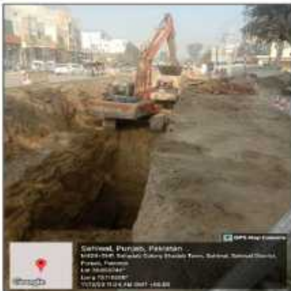
Picture 19: Pipe laying in progress at pakpattan road under LOT-4 SAHIWAL
