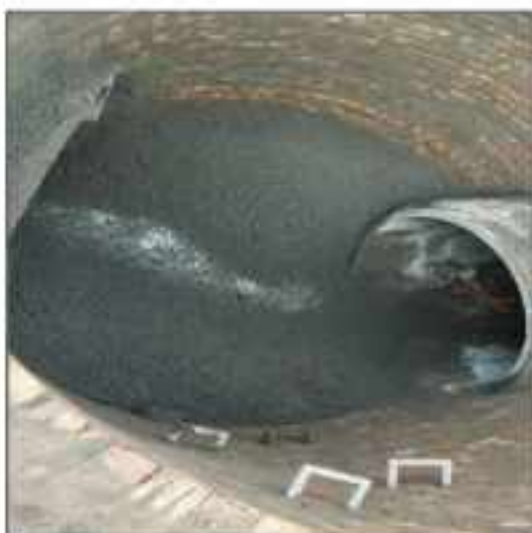
Picture 43: Benching is in progress at MH#60 KSR 66' Line LOT-1 Sialkot
