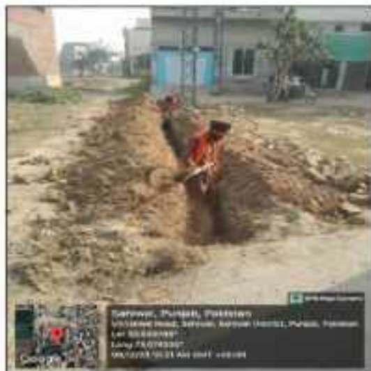
Picture 12: Laying of water supply lines under LOT-1 Sahiwal
