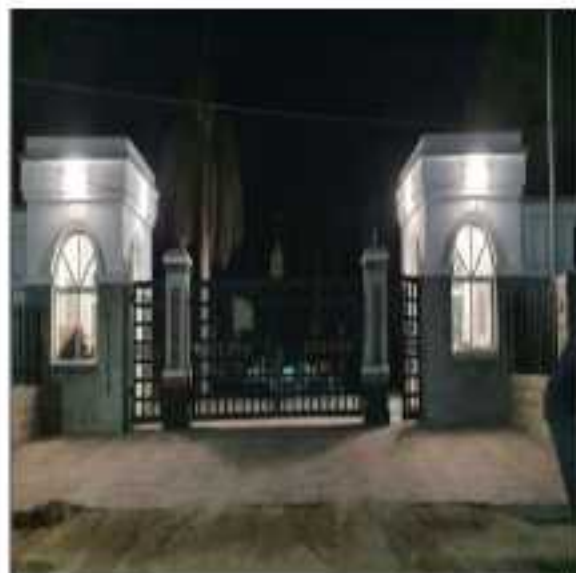
Picture 6: Lights of Security & Ticketing Rooms of Gulshan Iqbal Park
