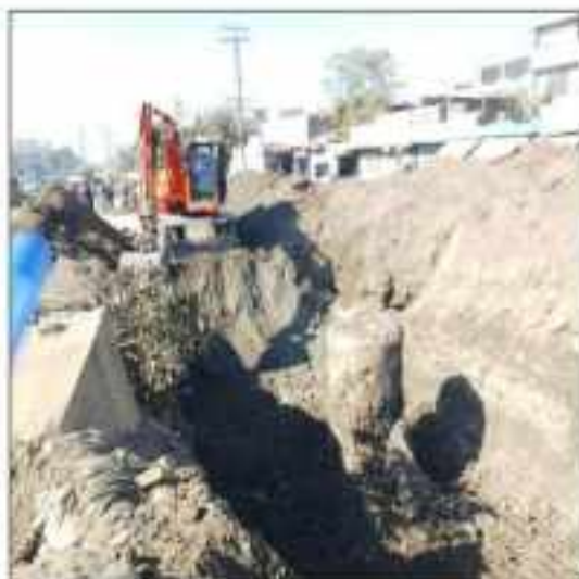
Picture 80: Excavation of retaining wall is in progress at flyover Sialkot.
