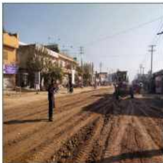
Picture 47: Restoration is in progress at Airport Road LOT-3 Sialkot.
