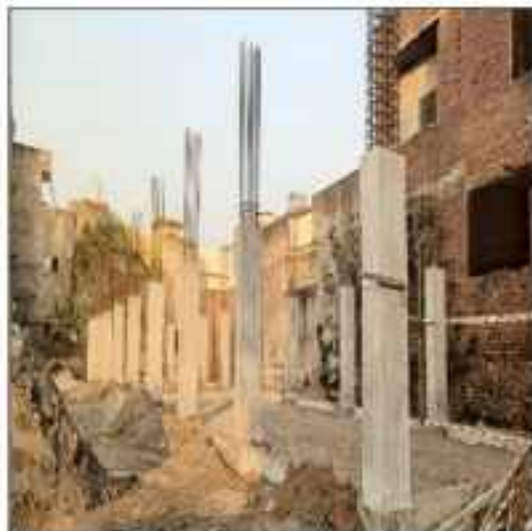
Picture 56: Column concrete is in progress at Iqbal town parking Sialkot.
