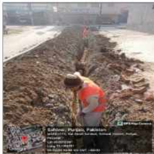
Picture 13: Restoration work under LOT-1 Sahiwal
