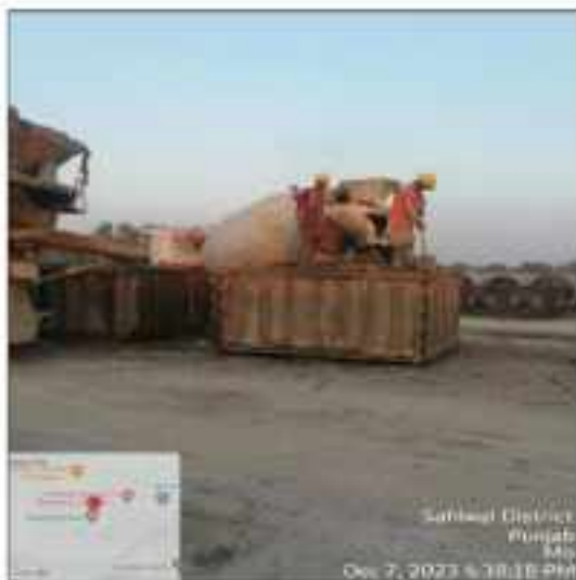
Picture 23: Pouring of conduit under LOT-3 is in progress.
