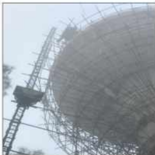
Picture 44: 1-50 Islamia College Water proofing OHWR#50 work in progress LOT-4 Sialkot.
