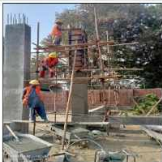
Picture 57: Columns concrete pouring is in progress at parking sheds.
