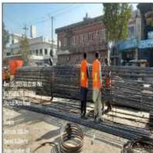
Picture 77: Steel cage fabrication is in progress at flyover Sialkot.
