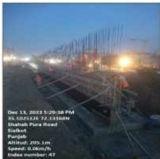
Picture 76: Retaining wall form work is in progress at flyover Sialkot.
