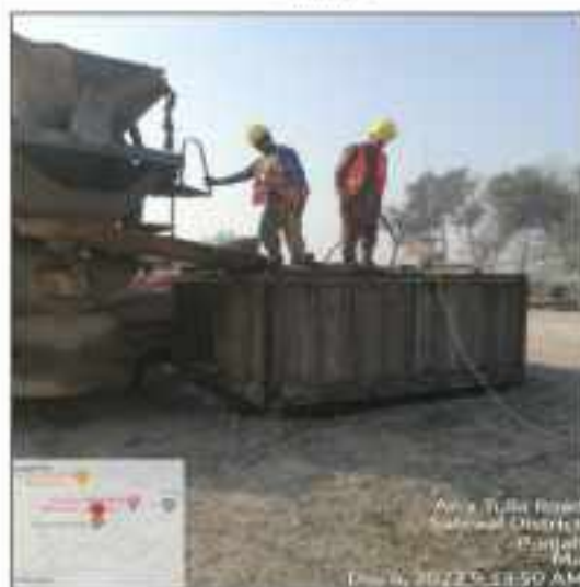
Picture 11: Concrete pouring of conduit under LOT-3 Sahiwal.
