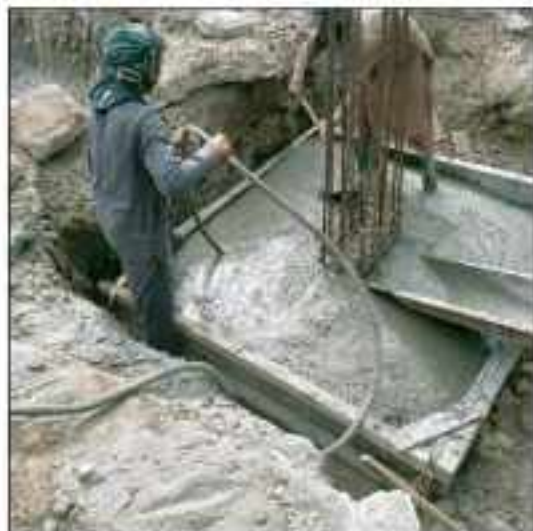
Picture 55: Work is in progress at Sahiwal Parking Shed.
