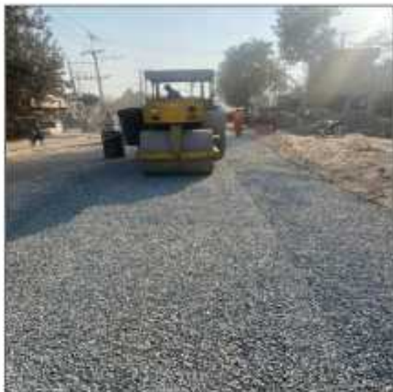
Picture 16: TST is in progress at Kacha Pakka Noor Shah Road LOT-2 Sahiwal.
