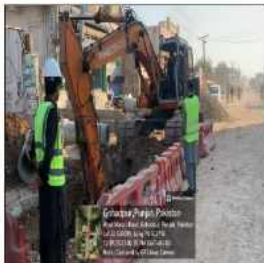
Picture 20: Excavation at Head Marala Road 21 LOT-1 Sialkot.
