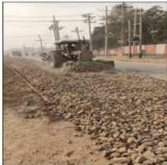
Picture 20: Restoration work LOT-2 Sahiwal is in progress
