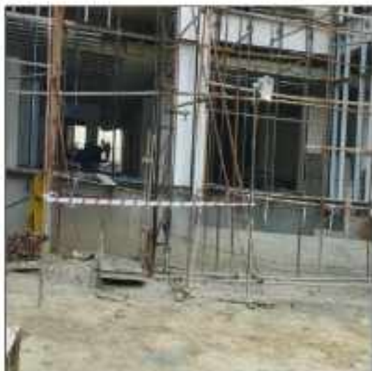
Picture 51: Shuttering view
