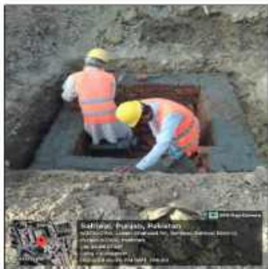
Picture 22: Construction of chamber is in progress under LOT-1 Sahiwal
