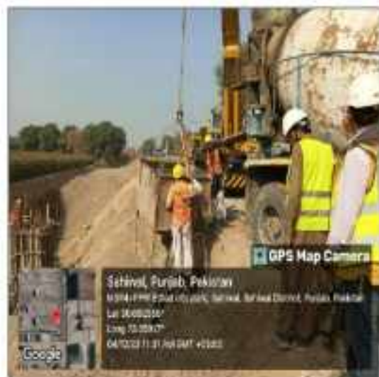
Picture 8: Manhole No.67 concrete pouring at small conduit site LOT-3 Sahiwal.
