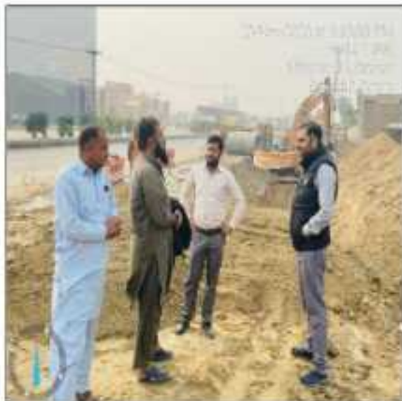
Picture 26: Work is in progress at LOT-4 48 DIA Sahiwal
