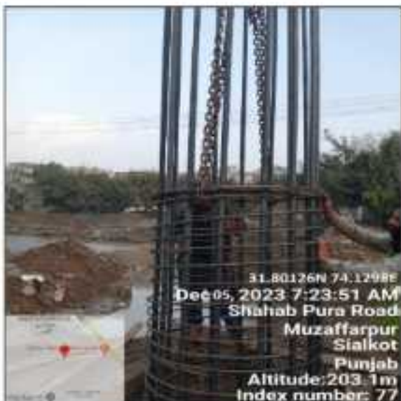
Picture 73: Cage lowering is in progress at flyover Sialkot.
