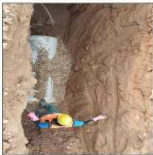
Picture 39: Pipe laying is in progress at line 3.9.1 Marala Rd -21 Line.
