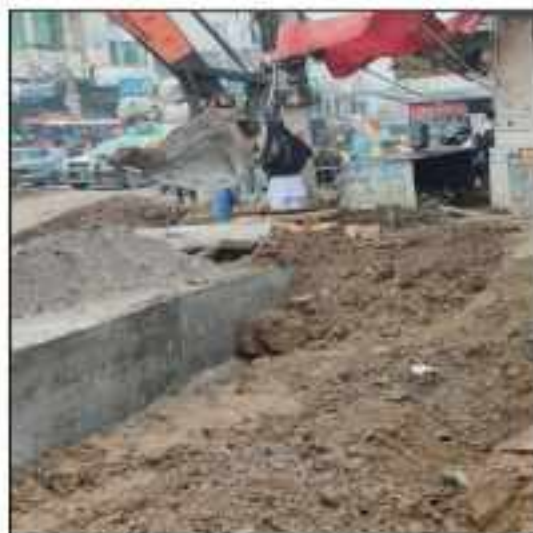
Picture 30: Gohad Pur Chowk drain back filling is in progress at LOT-2 Sialkot.
