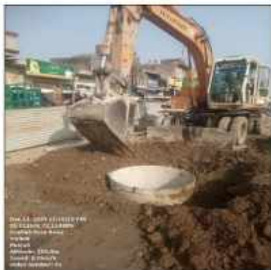
Picture 78: Pile excavation and layout is in progress at flyover sialkot.
