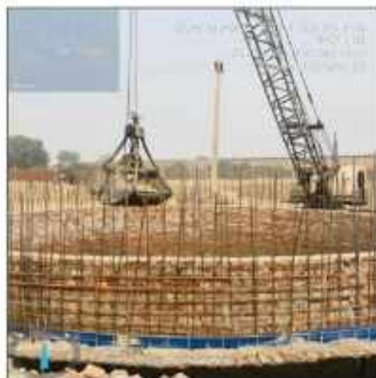
Picture 9: Work is in progress at LOT-4 Disposal Station.
