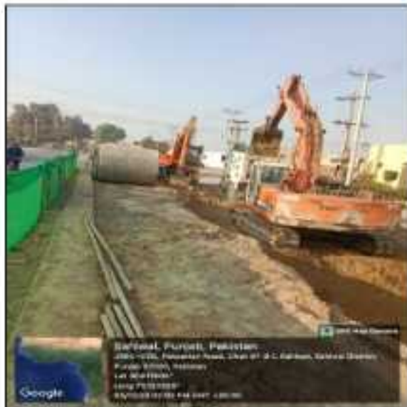
Picture 25: Laying of 72" DIA pipes under LOT-4 is in progress.
