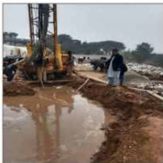
Picture 42: Supply well drilling in progress at P-55 LOT-3 Sialkot
