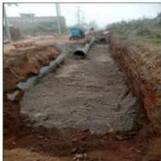
Picture 29: Bed dressing work is in progress at LOT-3 Sialkot.
