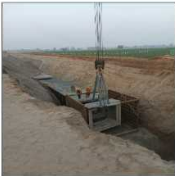
Picture 17: Laying of conduits are in progress under LOT-3 Sahiwal.
