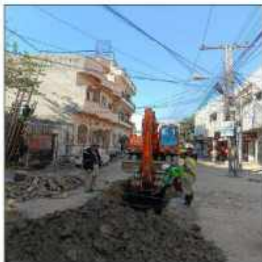
Picture 40: Excavation is in progress at Jinnah Street LOT-1 Sialkot
