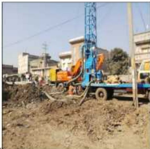
Picture 65: Drilling is in progress at flyover Sialkot.
