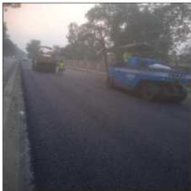
Picture 64: Laying of Asphalt at Iqbal Road is in progress.
