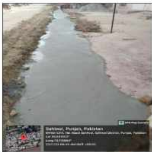
Picture 14: Restoration work is in progress at LOT-1 Sahiwal
