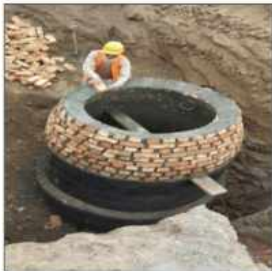
Picture 36: Brick masonry for MH 33, Marala Rd 42 nd pipeline, lot 1 Sialkot
