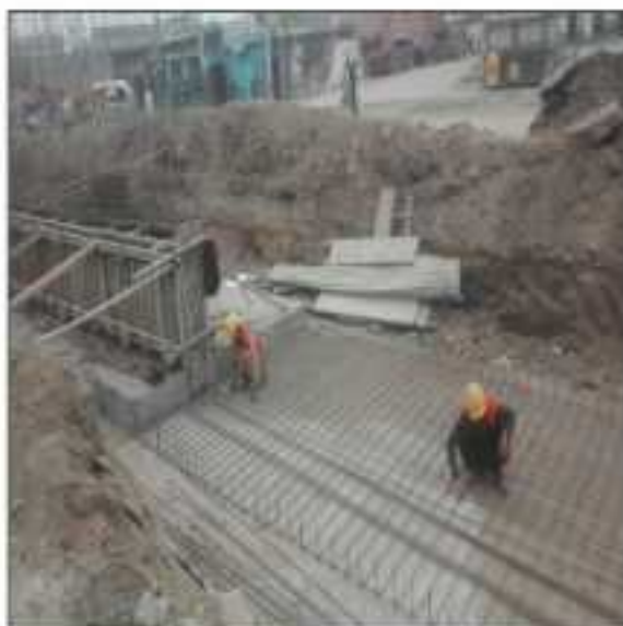
Picture 83: Reinforcement fabrication is in progress at retaining wall flyover Sialkot.
